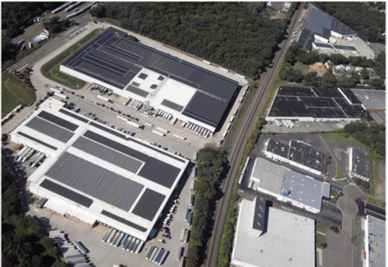
Pictured Above: Hall's Warehouse Corp. 501, 601 and Oak Tree Facilities with New Jersey's Largest Privately held Rooftop Mounted Solar Installations
